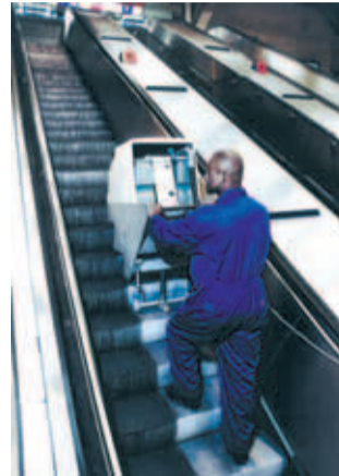
Escalator cleaning in-situ using the Rotomac 330
